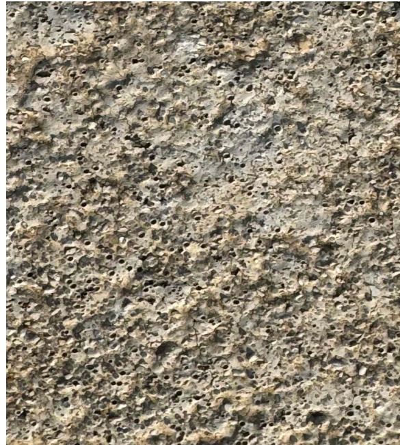
Figure 54 – Condition of the road marking as of 26 May 2025.
