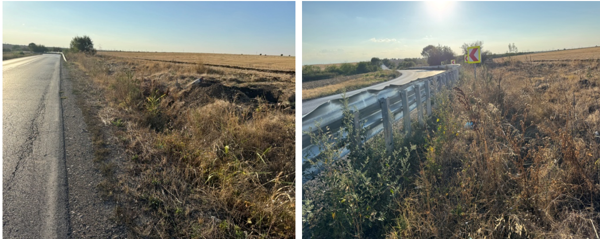
Figure 39 – Condition of the slopes in the studied section (direction from town Knezha to town Byala Slatina).
