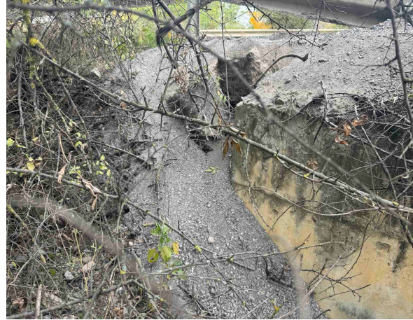
Figure 23 – Condition of the culvert at the road maintenance base, view from the north side.
