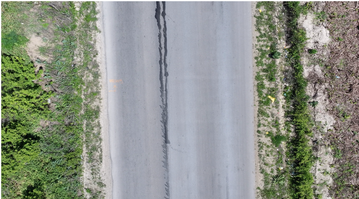
Figure 40 – Condition of the slopes, visualization from surveying performed by the EUCTP team in May 2025 using the remote sensing method.
