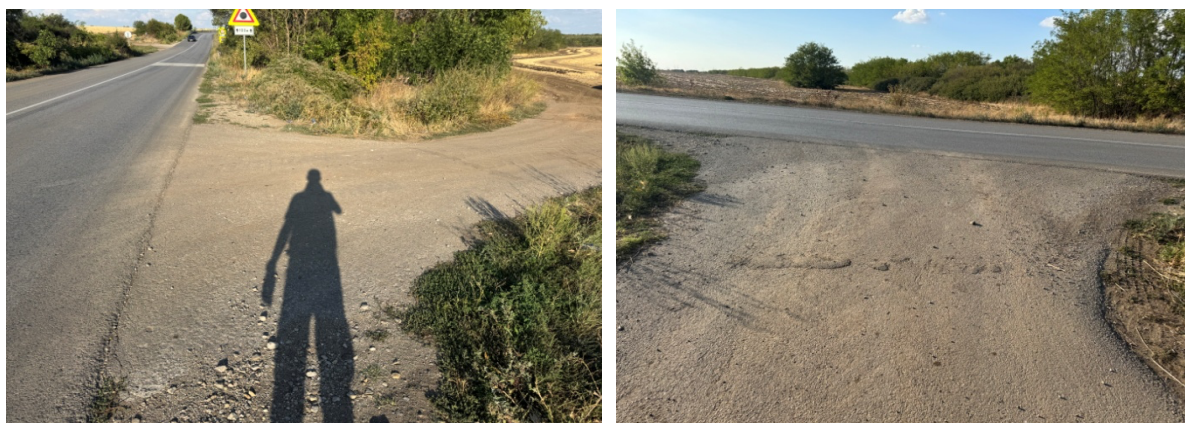
Figure 11 – Established the presence of asphalt pavement at the turn-off for the agricultural/forest road and the absence of road sign B2 on the right side in the direction from town Byala Slatina to town Knezha.
