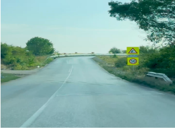
Figure 49 – Overall condition of the road marking as of September 2025, after the safety measures for the UKPTP were implemented.
