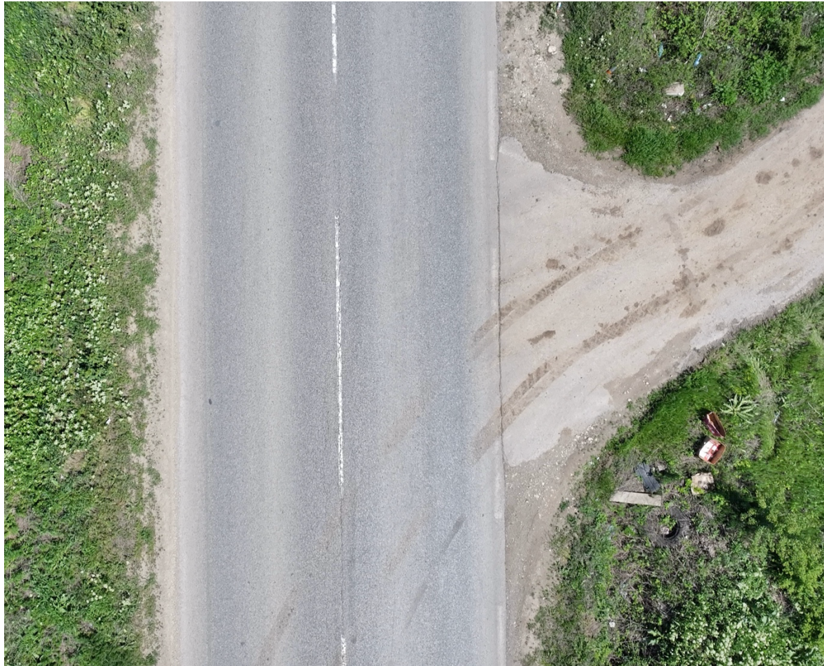
Figure 12 – Condition of the unregulated intersection between road II-13 and an agricultural-dirt road at km 65+717. Excerpt from surveying performed by the ECTP using the remote sensing method.
