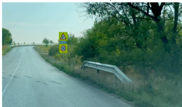
Figure 29 – Example of vegetation clearing behind the road maintenance base – right traffic lane in the direction of travel (town Byala Slatina → town Knezha).
