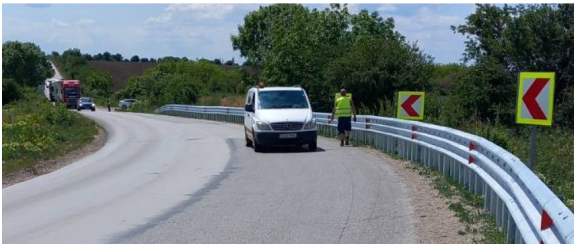
Figure 63 – Photo from the installation of the road restraint system on 20.05.2025. Source: https://api.bg/bg/novini/montirani-sa-novi-mantinel-na-put-ii-13-byala-slatina-knezha-pri-66-i-km-za-obezopasyavane-na-uchastuka-s-kontsentratsiya-na-intsidenti.html
