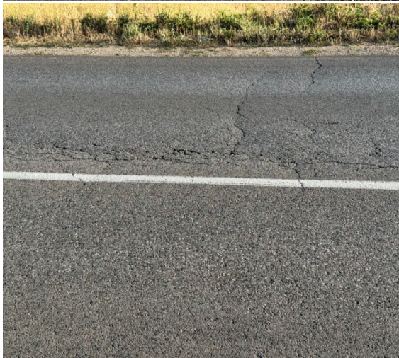
Figure 78 – Presence of mesh-like and block cracks in numerous zones.
