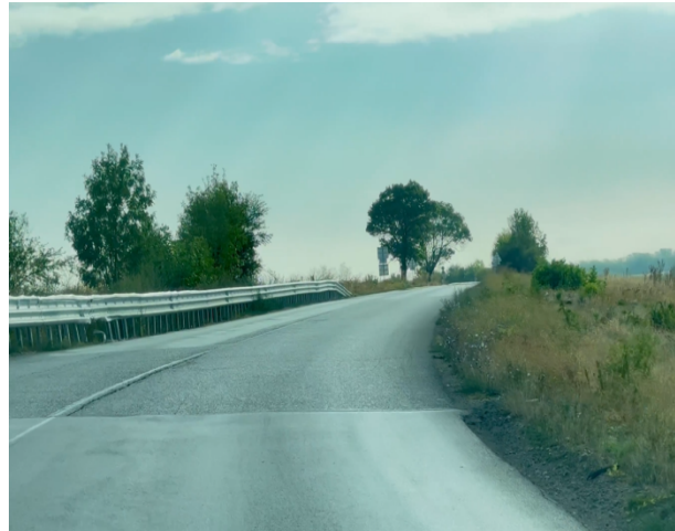
Figure 42 – General view of the traffic lane in the direction from town Byala Slatina to town Knezha.
