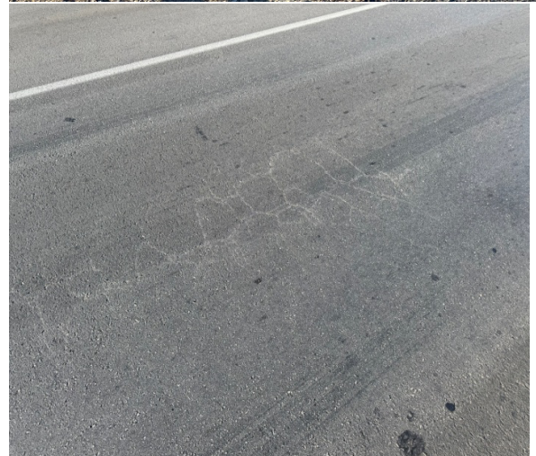
Figure 79 – Presence of mesh-like and block cracks in numerous zones.
