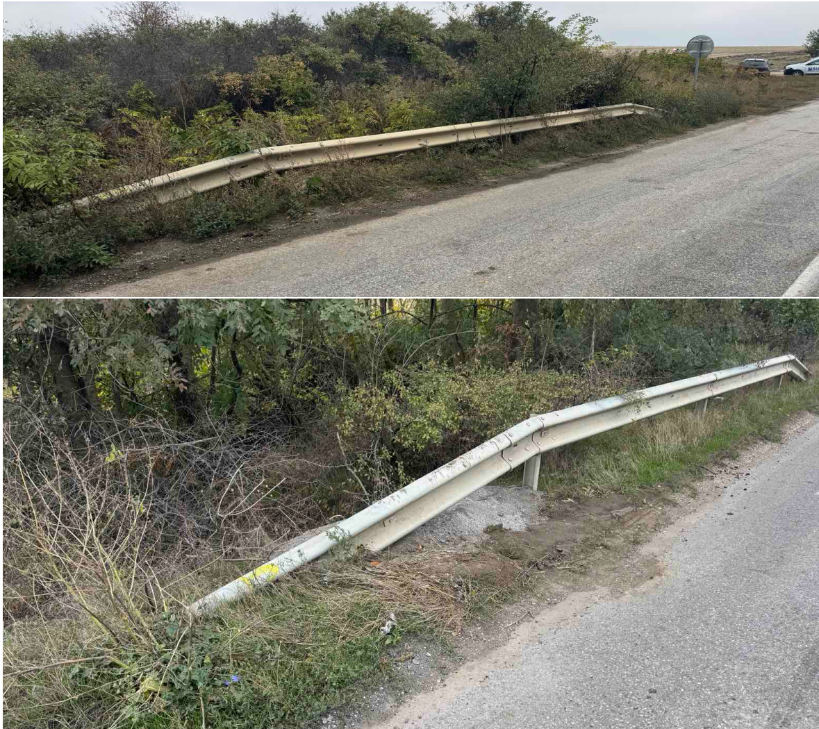
Figure 71 – Condition of the road restraint system on both sides of the culvert located at km 65+770.
