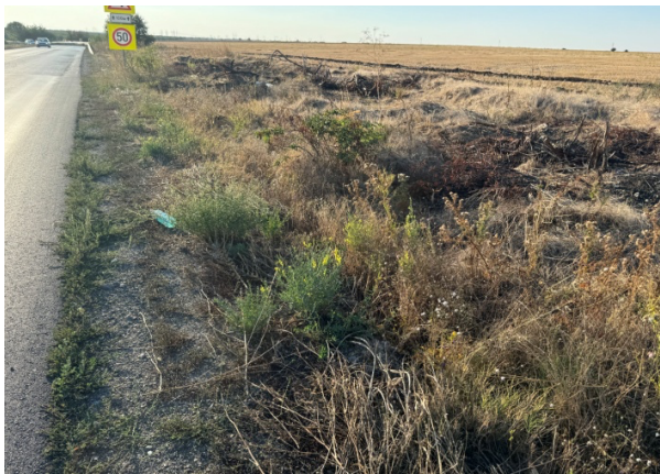
Figure 36 – Condition of the shoulder – right traffic lane in the direction of travel (town Knezha → town Byala Slatina).
