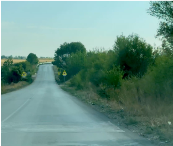
Figure 41 – General view of the traffic lane in the direction from town Byala Slatina to town Knezha.
