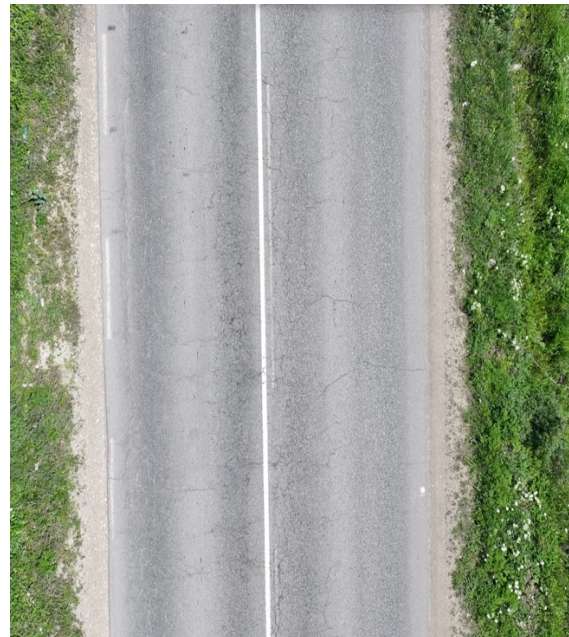
Figure 52 – Condition of the road marking as of May 2025 before the safety measures for the UKPTP were implemented – footage captured by the remote sensing method.
