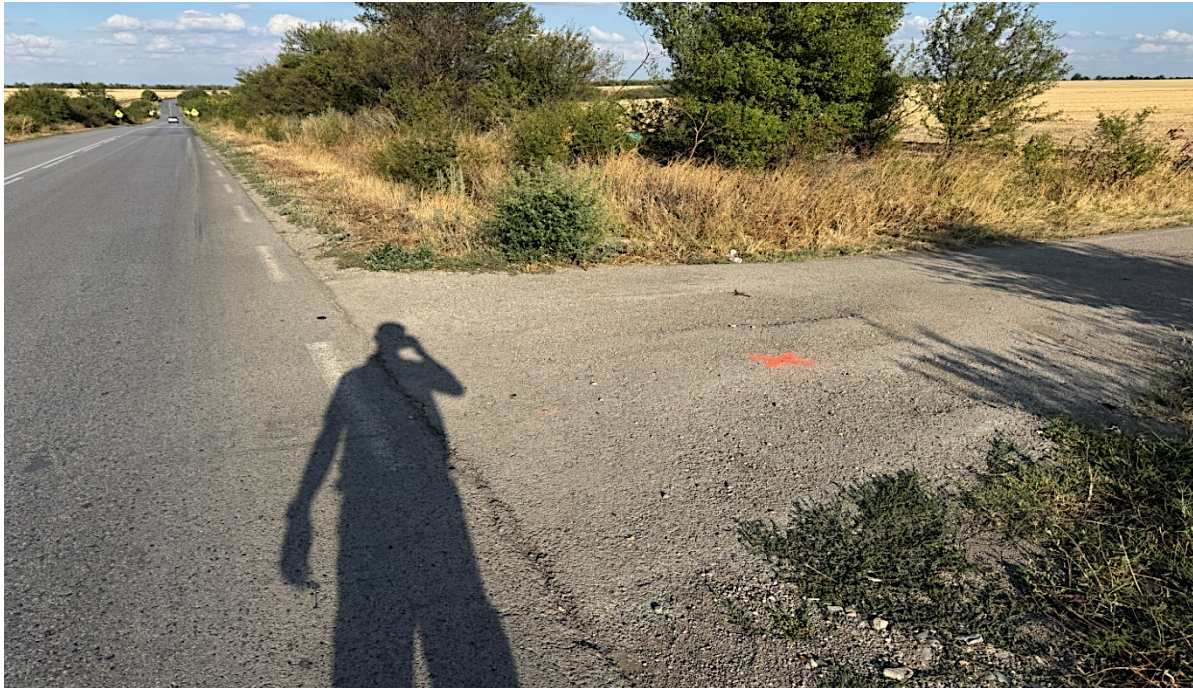
Figure 7 – Unmarked agricultural/forest road, located on the right side of the traffic lane in the direction from town Byala Slatina to town Knezha, at the beginning of the inspected section.
