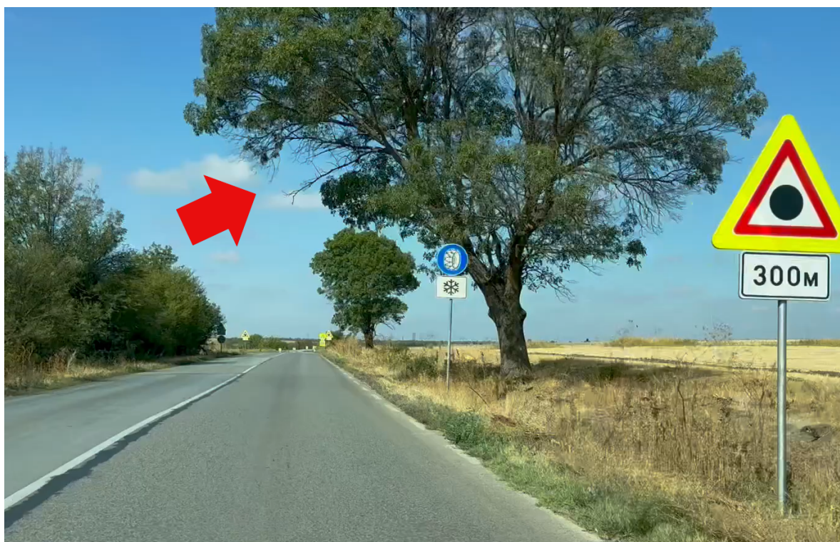
Figure 82 – On-site, a tree was identified with dried branches extending over the traffic lane.
