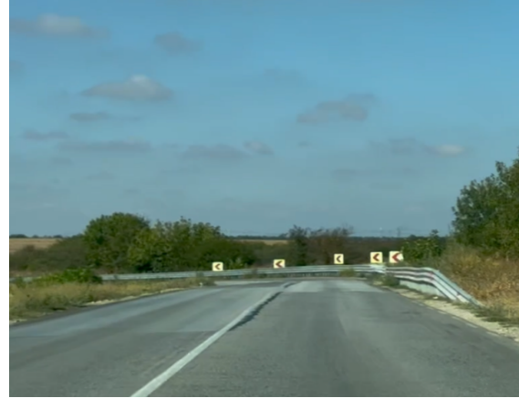
Figure 50 – Overall condition of the road marking as of September 2025, after the safety measures for the UKPTP were implemented.
